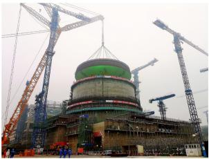
Figure 9. Dome Hoisting of Fangchenggang NPP Unit 4
