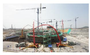
Figure 13. Concrete Pouring Site of Zhangzhou NPP Unit 2
