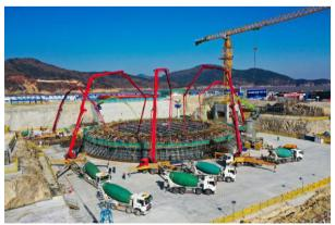
Figure 17. Concrete Pouring Site of San'ao NPP Unit 1
