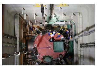
Figure 12. Three Shell Assembly of the HTGR NPP Demonstration Project (Primary Circuit Equipment such as Pressure Vessel, Hot Gas Duct, and Steam Generator are Connected)
